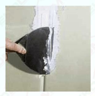
**DESCRIPTION**: Ekofix G9 is construction adhesive for plasterboards
